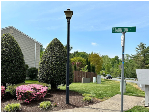
Typical street light
