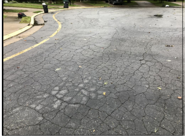
Typical condition of older asphalt surfaces
