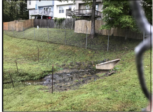
Retention pond culvert
