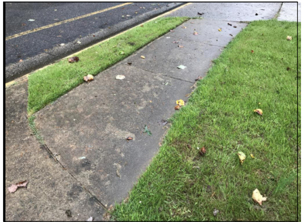
Typical condition of concrete sidewalks
